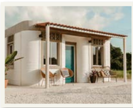
3D-printed home in Tabasco, Mexico. icon build.com
